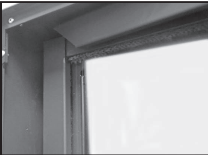
Figure 56: Installing top trim.
