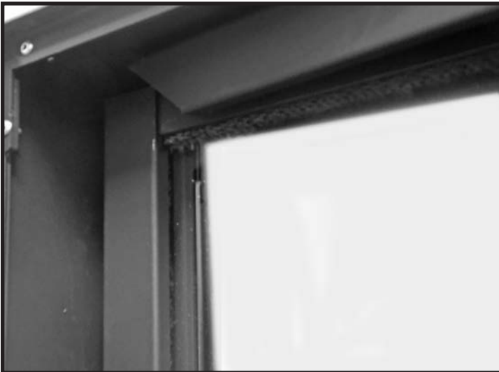
Figure 56: Installing top trim.
