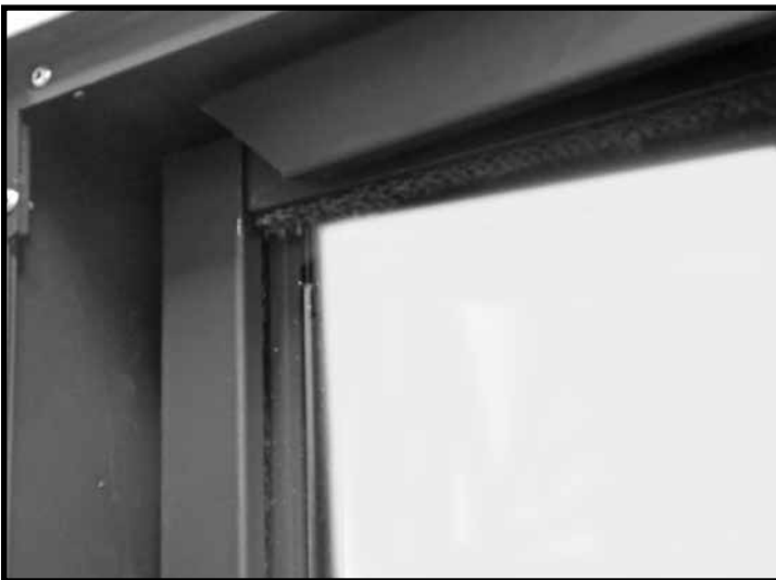
Figure 52: Installing top trim.
