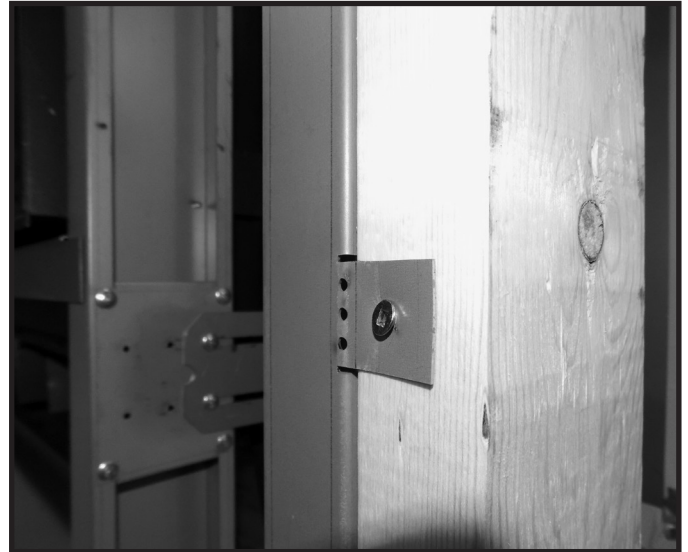
Figure 17: Attach tab to wood framing.
