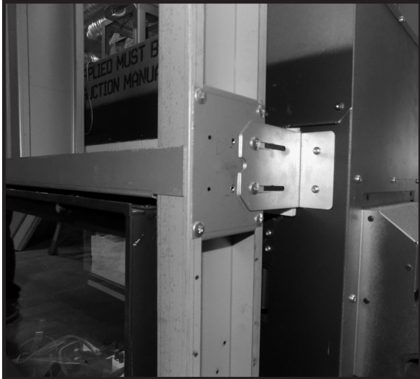
Figure 16: Framing bracket positioning.
