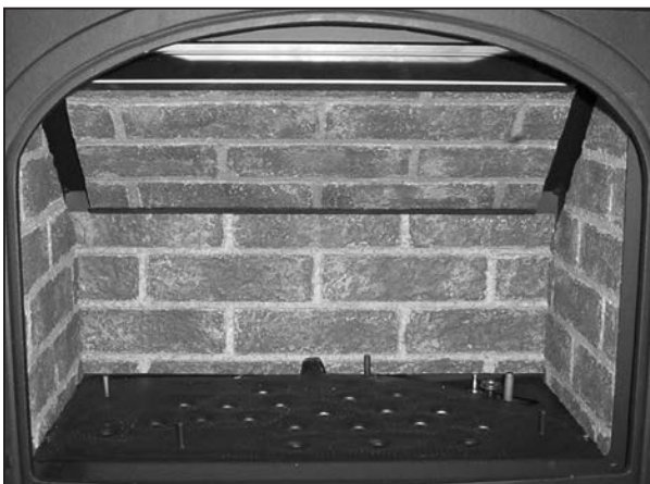
Figure 64: Side brick panels in place.
