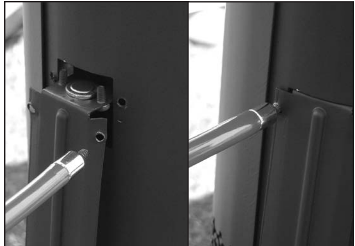
Figure 48: Spill switch installation.
