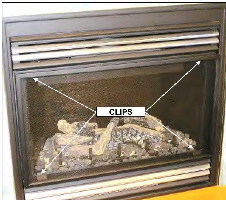
Hook Lower Clip onto glass door frame.
