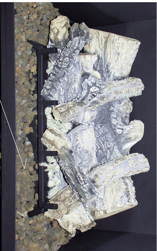
Step (10) Place crushed rocks onto firebox bottom. (NOTE: Do not place crushed rock onto burner tubes)
