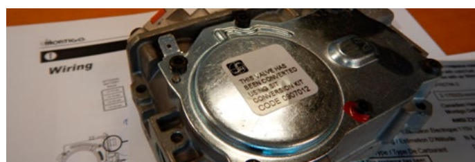
Figure 13.k Conversion label on valve
