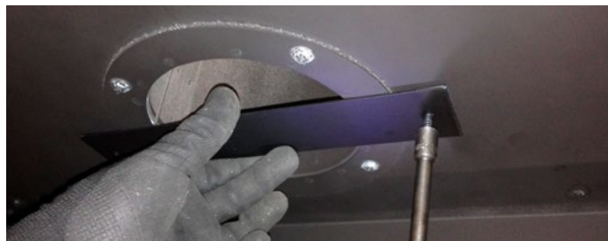
Figure 8.b.c Restrictor plate Installation
