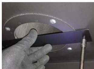
Figure 8.b.c Restrictor plate Installation
