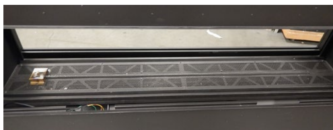
Figure 25.g Insert pilot cover/door/screen
