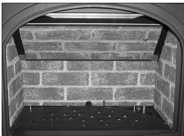
Figure 63: Side brick panels in place.
