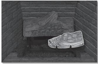
Figure 79: Log Set Installation - Step 2
