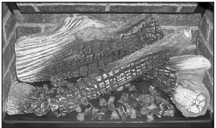
Figure 72: Log Placement with Rock Wool & Embers.
