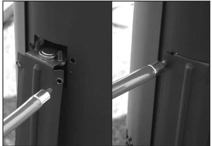
Figure 62: Spill switch installation.
