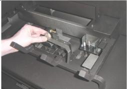
7 Remove the control panel to access the gas control valve. The stepper motor (adjustable regulator) has an installation sheet included with it – make sure to follow all of the directions. Place the stepper motor on the gas control valve (see Figure 1) – <u>MAKE SURE IT IS CORRECTLY ORIENTED</u>. Secure using the screws included with the motor (see Figure 2) – tighten to 25 Lb-inches. Leak test this area after installation to verify proper installation.
