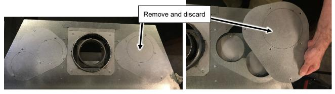
2. Remove the (4) screws that secure the two circular cover plates on the next layer of the fireplace. Carefully remove the two plates.
