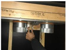
7 Remove the knockouts from the top of the fireplace. Use snips or diagonal cutters to snip the tab on the knockouts. Press on the far side away from the tap to pop the edge of the knockout upward.
