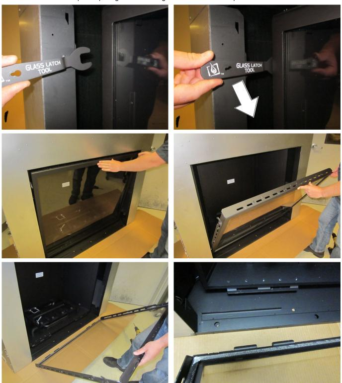
Installing the Firebacks
