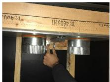
7 Stretch the included flex to its maximum length. Measure the distance between the starter collars on the fireplace and the inlets on the convection manifold. Cut the flex to the appropriate length and install between the fireplace and the manifold. Secure using (3) screws at every connection and seal the joints with silicone caulk or aluminum (U.L. 181A-P) tape.
