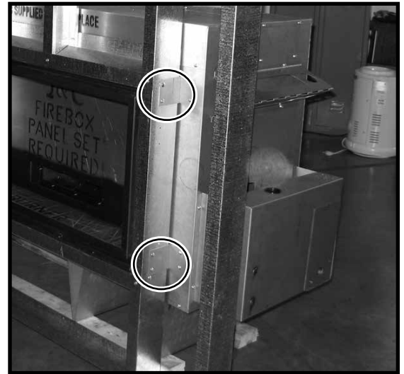
Figure 18: Framing bracket fastening points.
