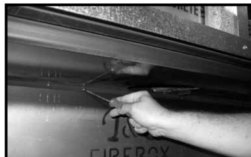
Figure 37: Securing top porcelain panel.
