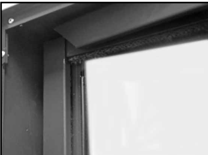
Figure 80: Installing top trim.
