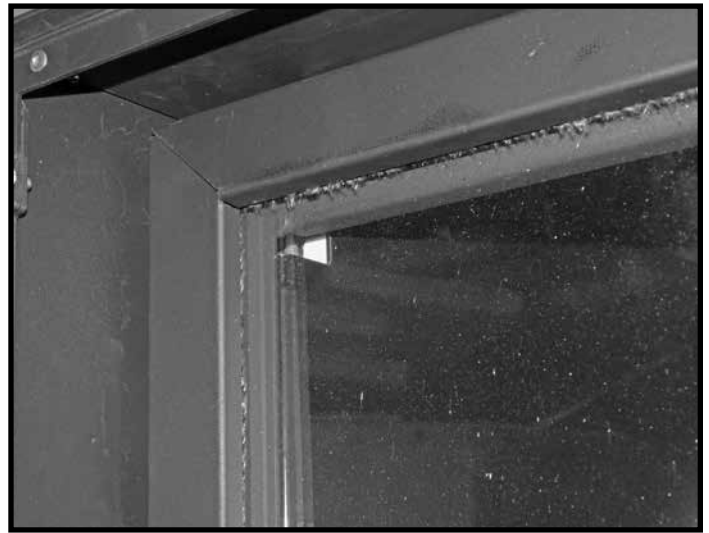
Figure 81: Top trim in place.
