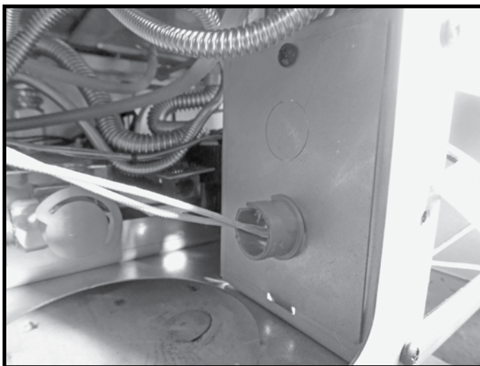
Figure 89: Threading wires through knockout.
