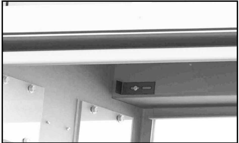
Figure 74: Panel retainer clip.
