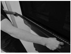
2. Lift up on the barrier screen assembly until the top brackets are clear of the tabs on the glass frame assembly. Direct the top edge of the barrier screen forward. Lift the bottom tabs out of the brackets on the bottom of the glass frame assembly and remove the barrier screen from the fireplace.
