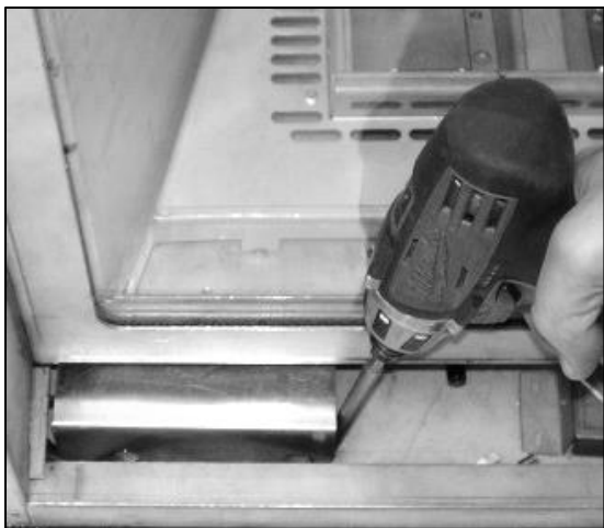
Power Vent Control Module Mounted inside fireplace.
