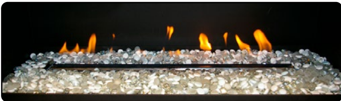
Figure 21.b Completed firestone installation
