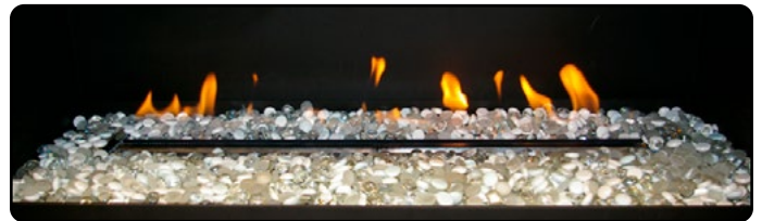
Figure 21.b Completed firestone installation
