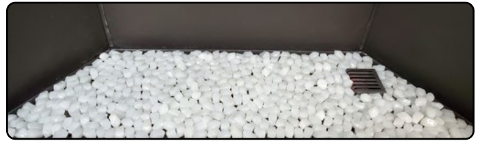
Figure 24.bb Completed firestone installation
