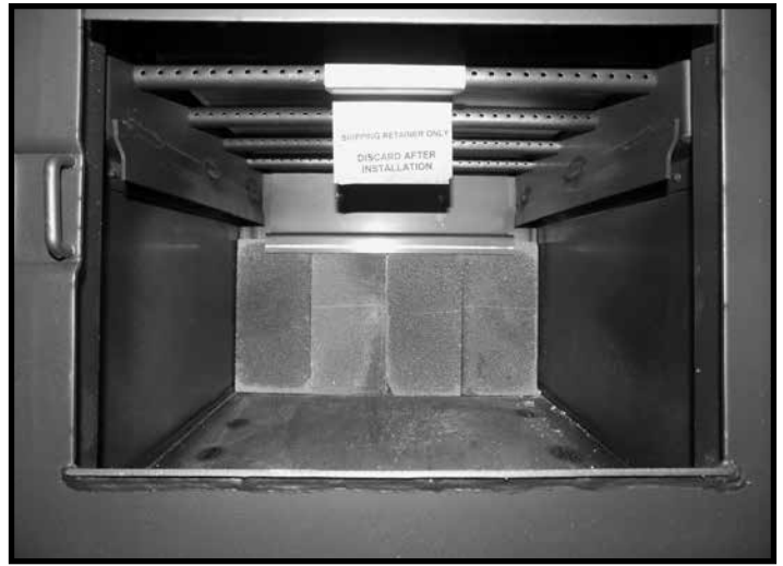
Figure 13: Bricks against rear wall.jpg
