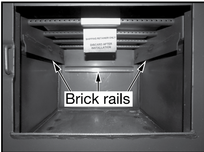
Figure 19: Firebox and brick rails.
