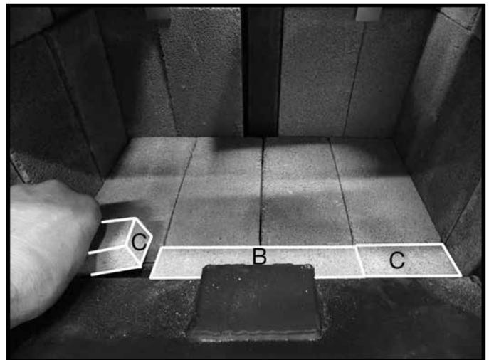
Figure 25: Narrow front bricks in place.
