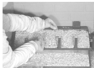
Figure 7 Placing Rock Wool
