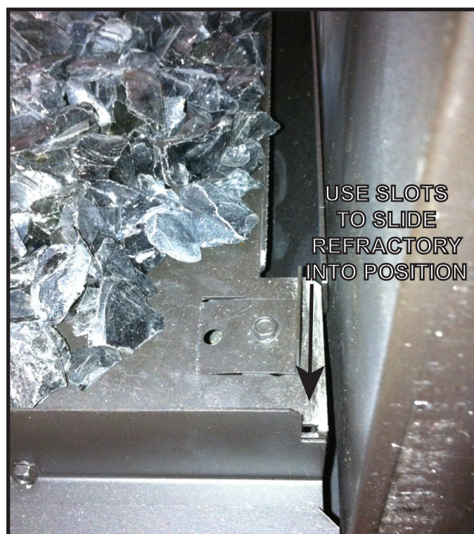
Figure 9.7 Install Refractory
