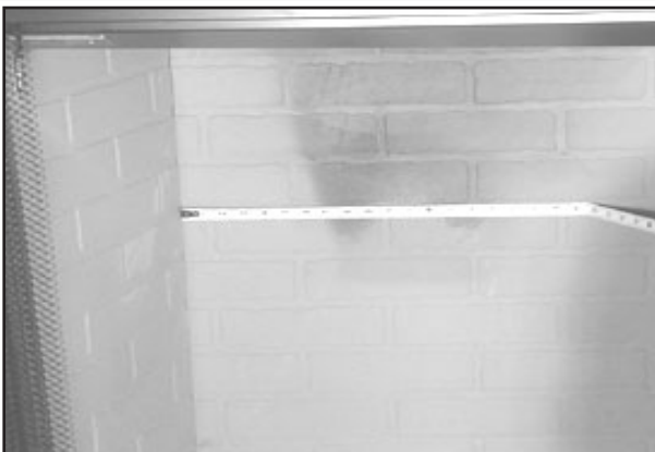
Figure 2.1 Measure Firebox
