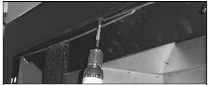
Figure 3.9 Removing the Screen Rods
