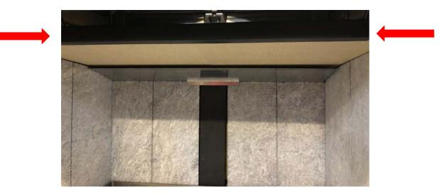
Photo 8. Baffle guard installed.
