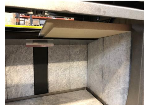
7) Install the right side vermiculite baffle into the firebox, as shown below.
