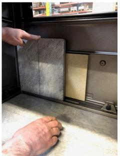
Photo 1. Insulation panel placed behind left rear refractory stone.
