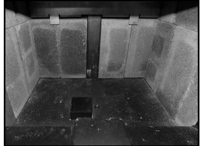
Figure 34: Firebox floor with ash dump.
