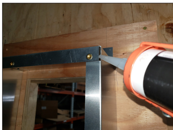
FIGURE 2.6 Appliquez le scellant silicone aux coins
