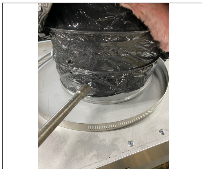
FIGURE 2.14 Screws in Inner Liner
