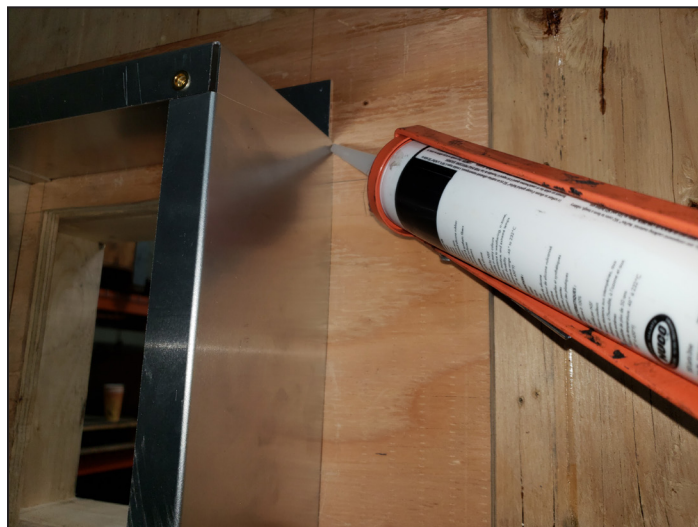
FIGURE 2.7 Silicone Perimeter
