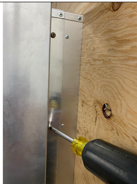
FIGURE 2.4 Retirez le couvercle
