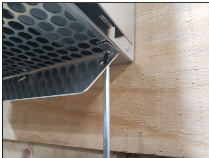
FIGURE 2.16 Vinyl Siding Shield Installed
